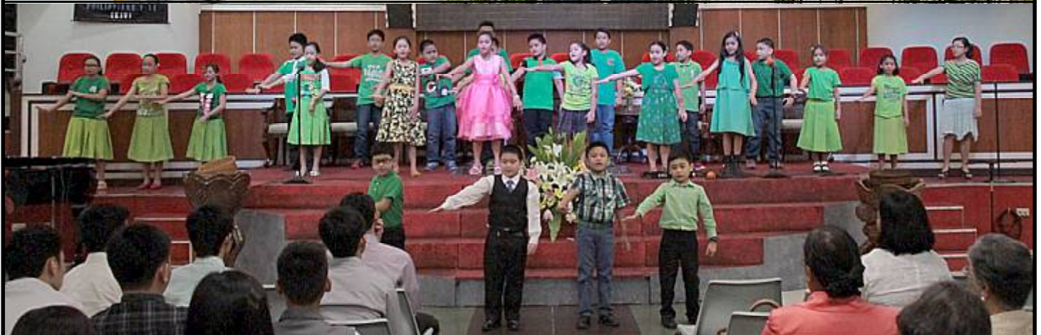
Top photo shows the steel structure of the Lighthouse Events Place nearing completion as the BBFPI1953 National Fellowship Meeting approaches to just four days away. Lower photo, the Lighthouse Psalters present their choral recitation last Sunday night.
